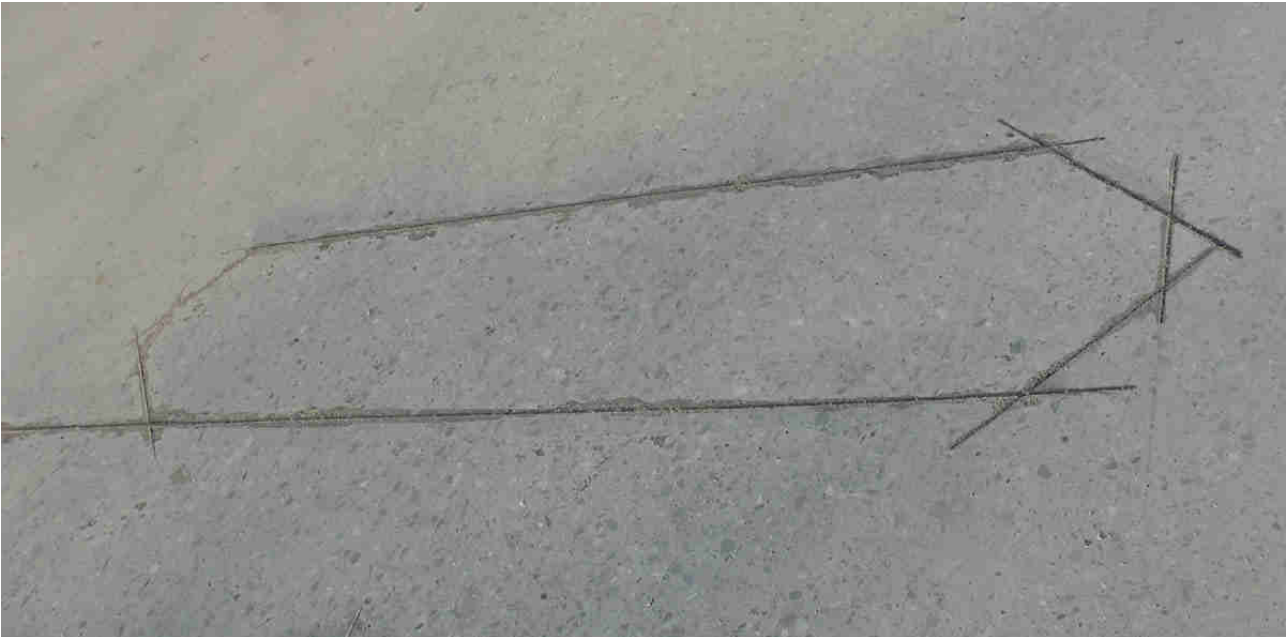
Induction loop cut into a concrete road
